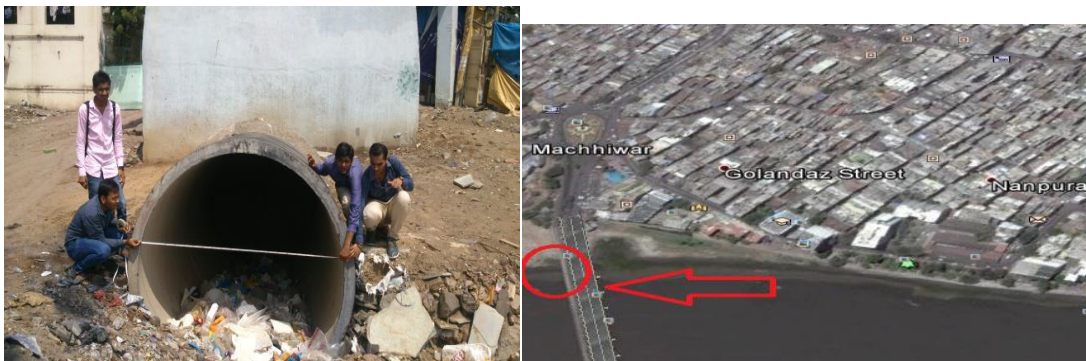
Figure.6 L6 Flood gate, U/S of Makkai Bridge
