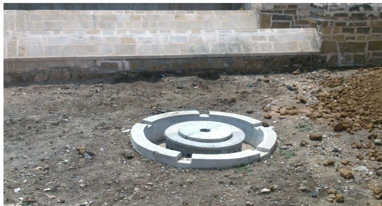
Figure.24 Construction of ground recharge well
