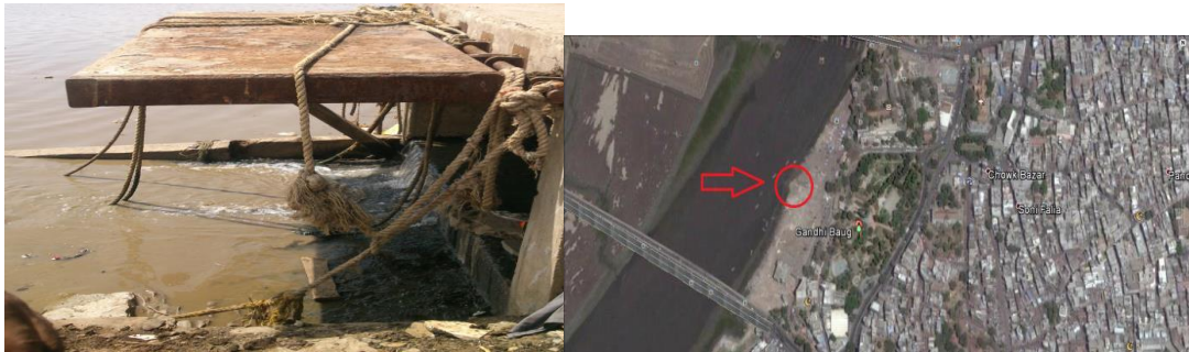
Figure.5 L5 Flood gate, Nr. Gandhi Baug
