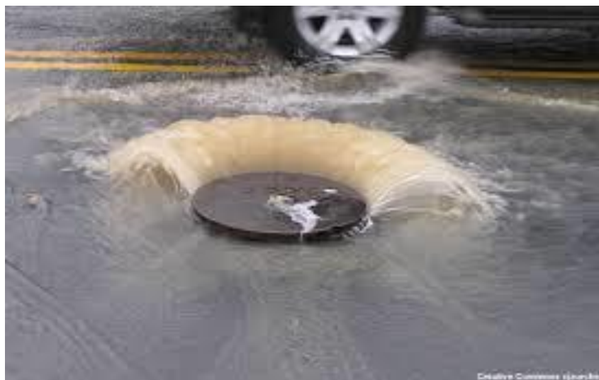
Figure.3 Critical water logging due to storm water back flow(2013)
