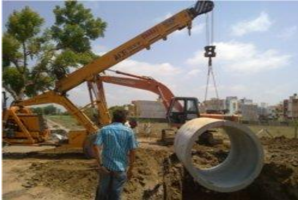
Figure.29 Storm water pipe installation
