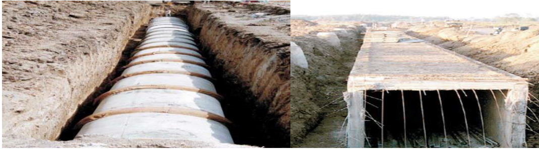
Figure.1 Construction of Storm water drainage line, Surat (Patel 2009)
